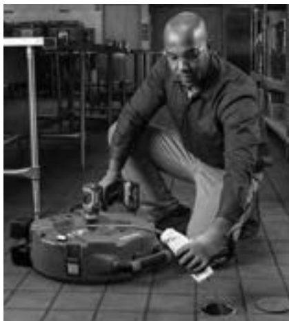
Figure 13 – Applying Lubricant to the Cable Sheath
